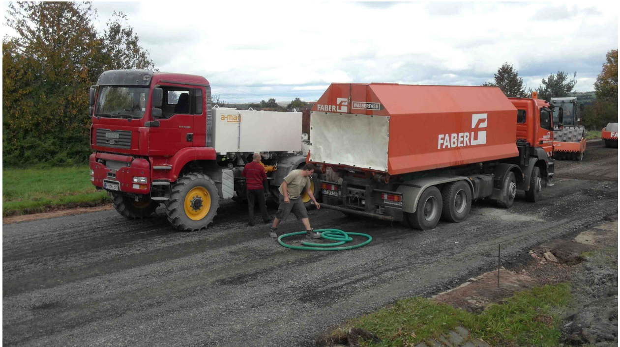
a-mag roll off-tank AT 23 with a capacity of 23 m 3 fills the 8 m 3 tank of the MFT MX®.
